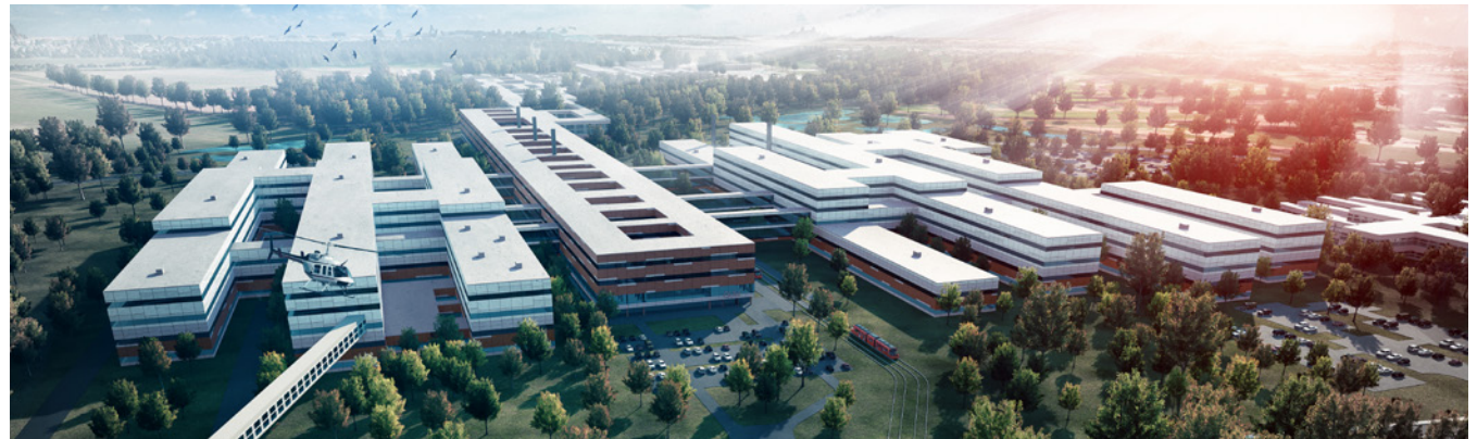
Symetri, part of the Design Management division, is providing Naviate Nexus software to the new Odense University Hospital (OUH), one of the largest construction projects in Denmark. Naviate Nexus streamlines dataflows and insures every contractor accesses the same information, a necessity for setting standards from a sustainability perspective, while making tracing materials simple and cost efficient.
